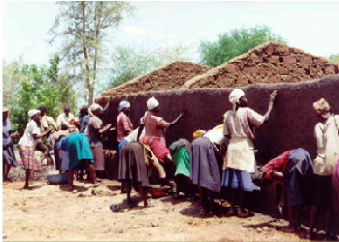
Figure 4: Women plastering mud rooms using mud mixed with aqueous extract of Parkia biglobosa fruit husk (Source: Margaret Shao) [5]
